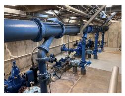
The pumping building has 6 pumps that supply water to residents and fill offsite holding tanks and the water tower on Miami Avenue. See picture at left.
